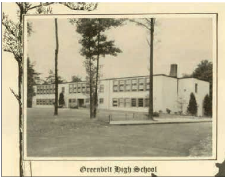
A photo of the 1938 building printed in the 1940 Greenbelt High School yearbook
